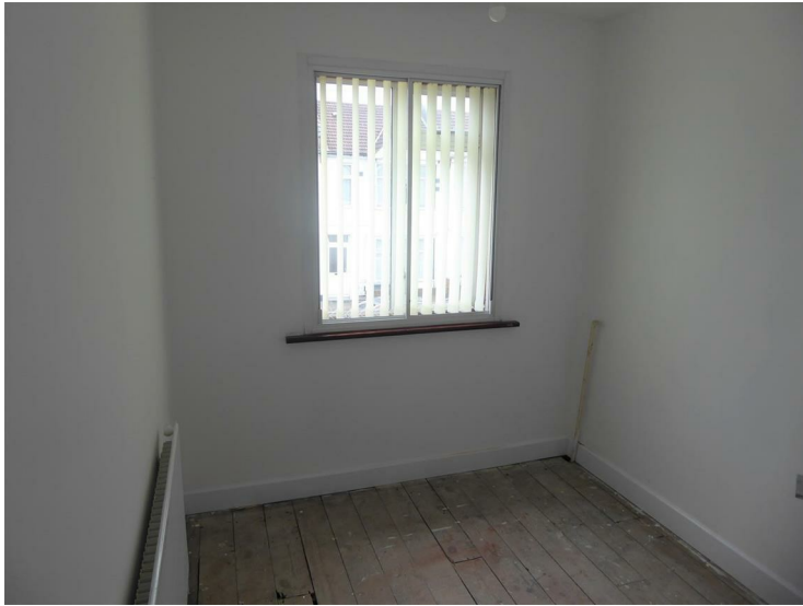
Front aspect double and secondary glazed window.
